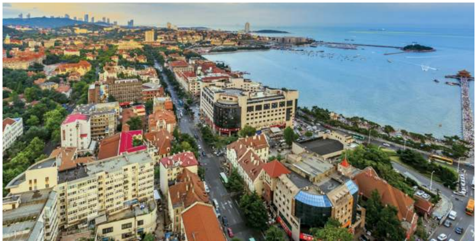
TOP: In 2013, Yanmar duplicated its Biwa diesel engine factory in Qingdao to meet sales demands ABOVE: Qingdao, China
