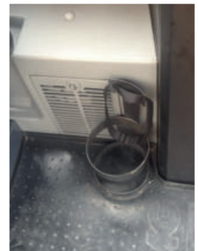
The fire extinguisher was originally intended to be fitted to the A-pillar, but this new location makes access to the AC filter impossible!
