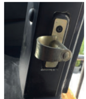
The finish of this recess takes me back to my days as a trainee joiner, when we occasionally used the expression, "It'll do for the lads"
