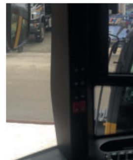
The bulging cabling behind this cover not only looks atrocious, but reduces visibility through the front windscreen. Another run of cable literally cut a corner and obscured the view to the ground at the left-hand side
